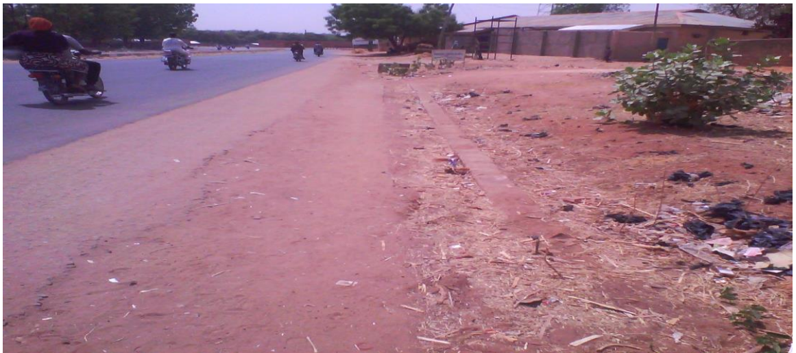
Plate 3: Drainage Blocked and Filled up (Site 3)
