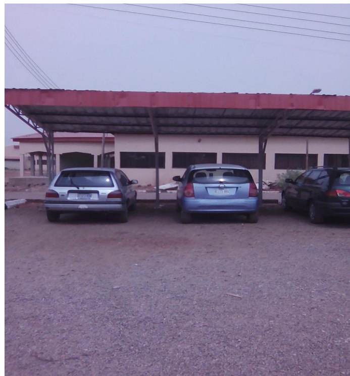
Figure 2.2: A view of a cantilever type car parking bay at the College of Engineering.
