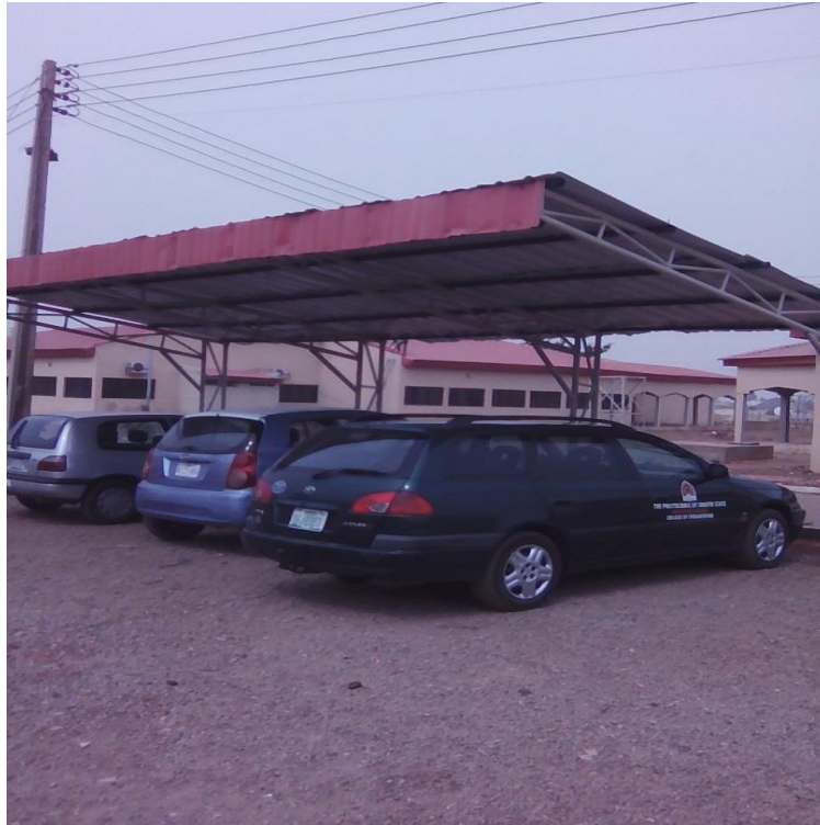
Figure 2.1: Car Park constructed at the College of Engineering
