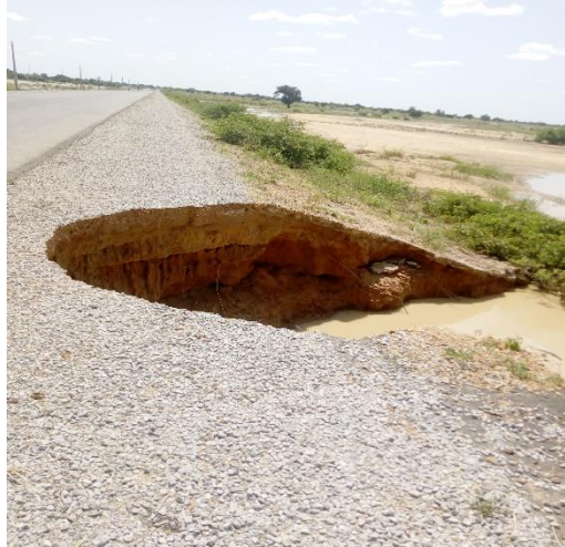
Plate 1: Washed away Road at Isa L.G.A. Plate 2: Road under threat of being washed out at Sabon Birni L.G.A.
