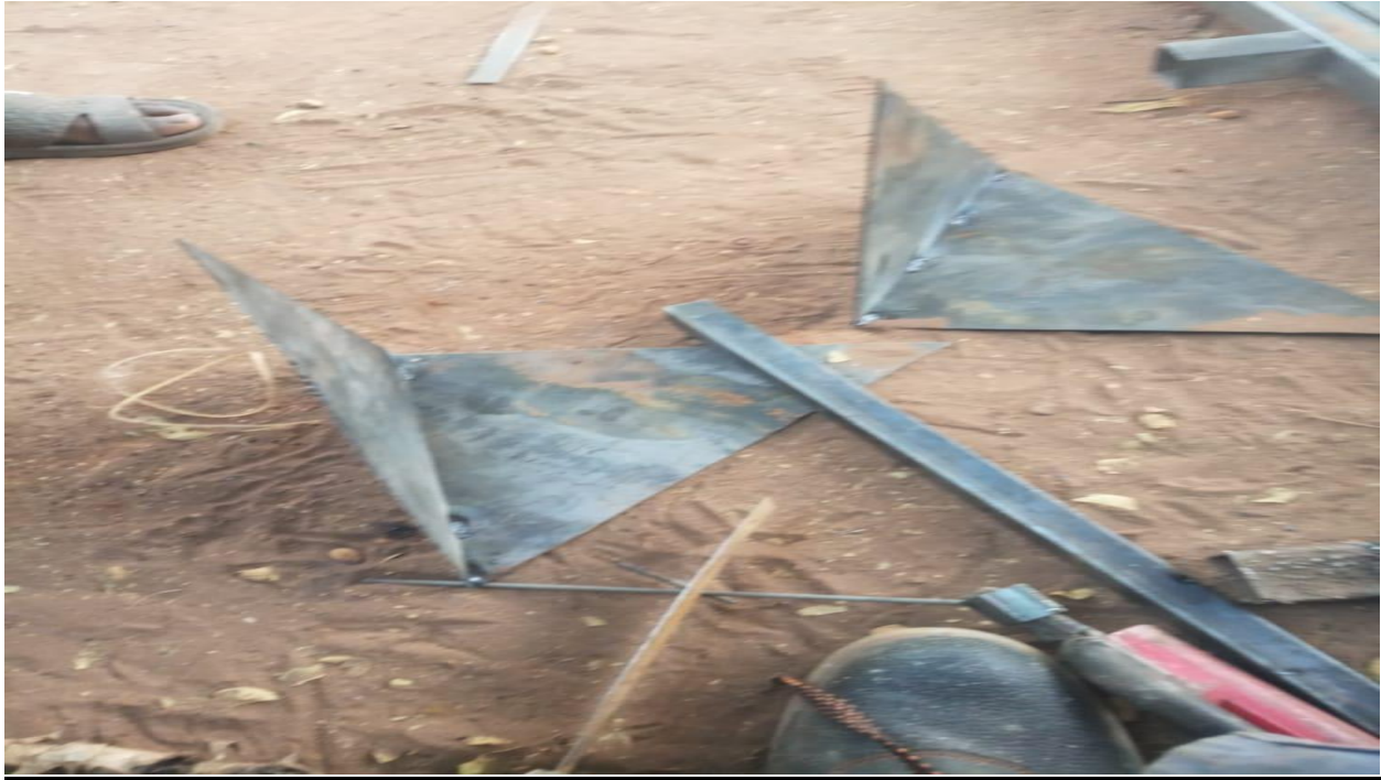
Plate 2: Joining/Connection of sheet metal for chimney construction in progress
