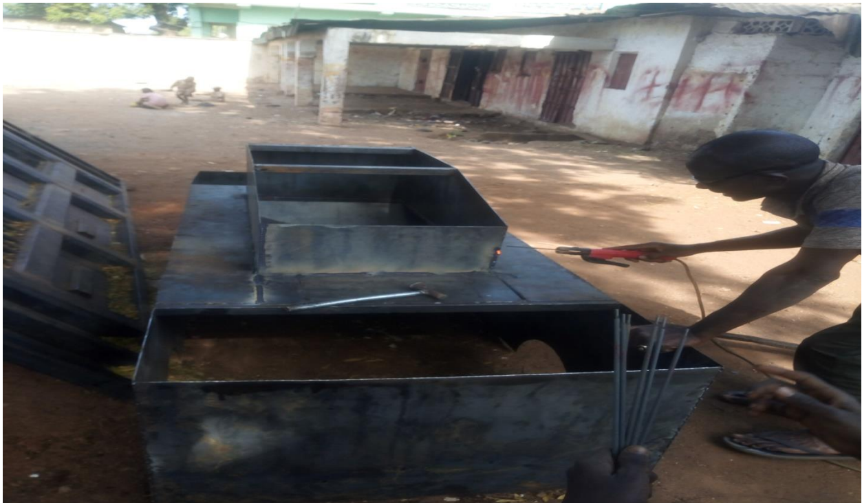
Plate3: Construction of the Incinerator in progress
