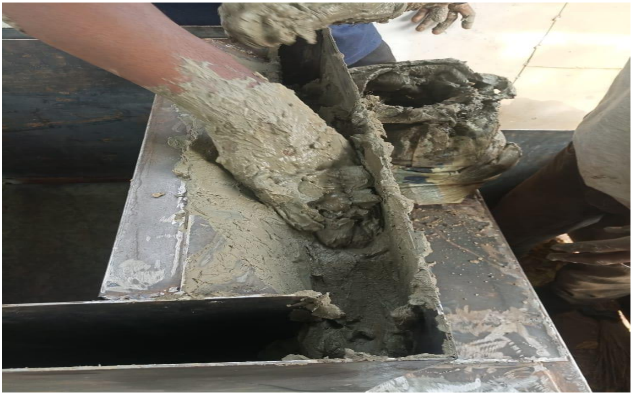
Plate 5: Lagging of combustion chamber with clay material in progress
