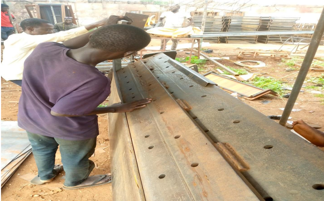
Plate4: Metal cutting and bending work cont.
