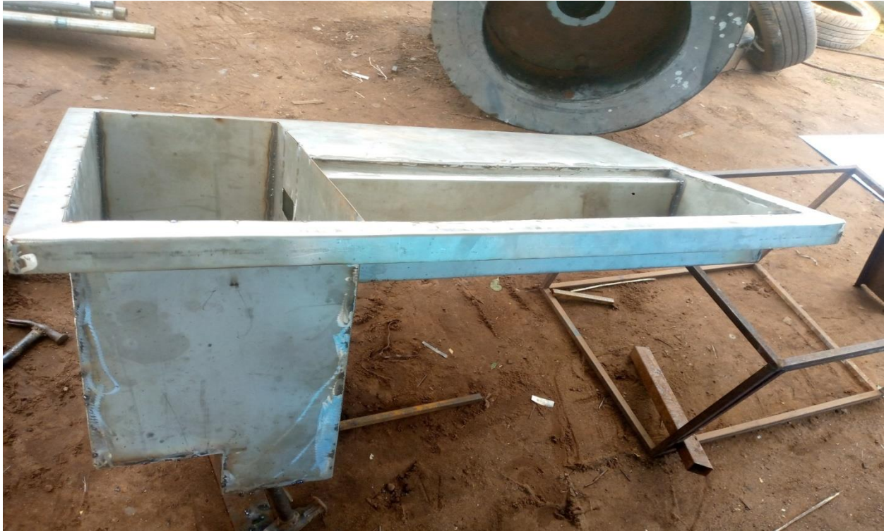
Plate8: View of an upper part of the fabricated hydraulic bench connected with welding.
