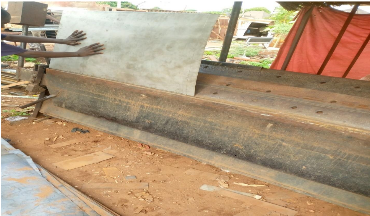
Plate5: Metal bending process cont.
