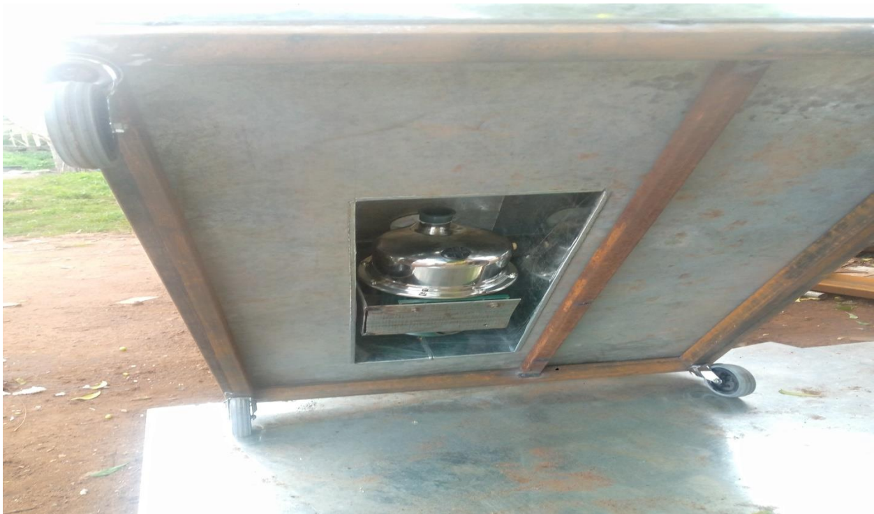
Plate17: Electric motor (1hp Centrifugal pump) fixed at the bottom of the hydraulic bench for pumping
