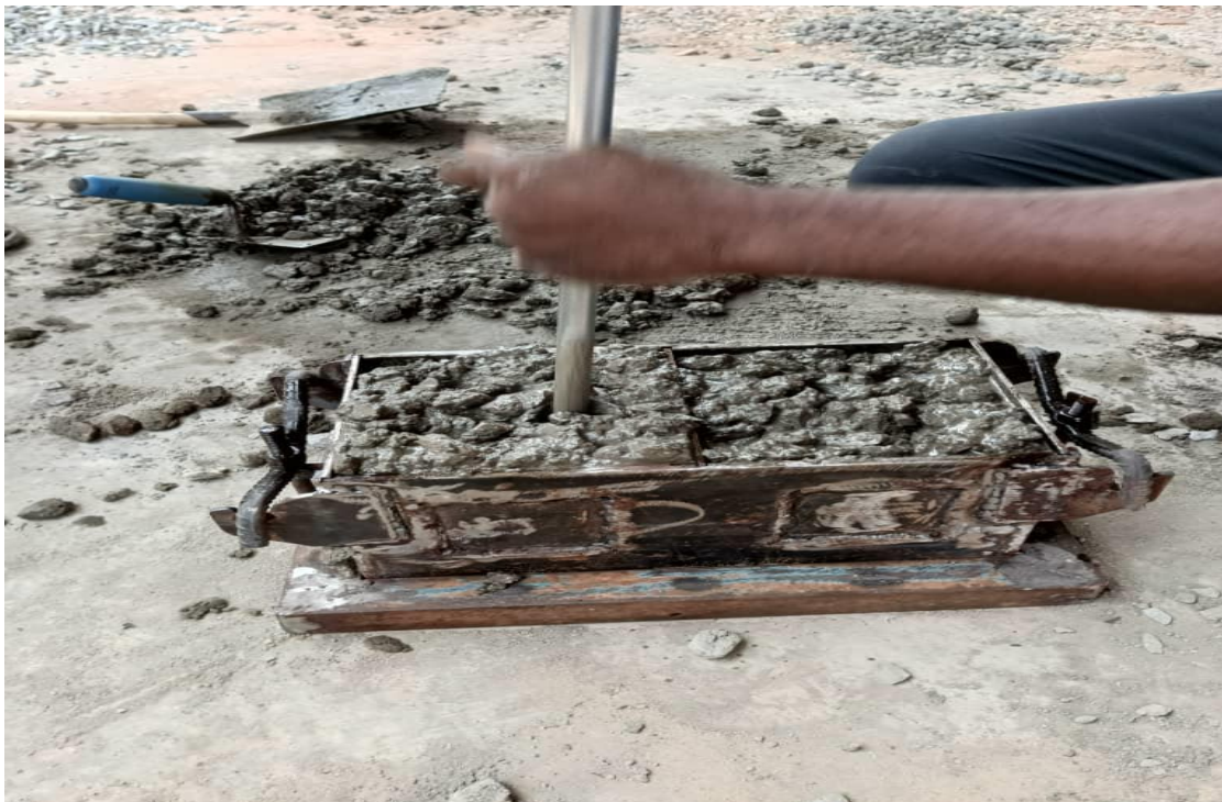
Plat 11: Hand compaction of concrete with the fabricated mold to produce a cube.
