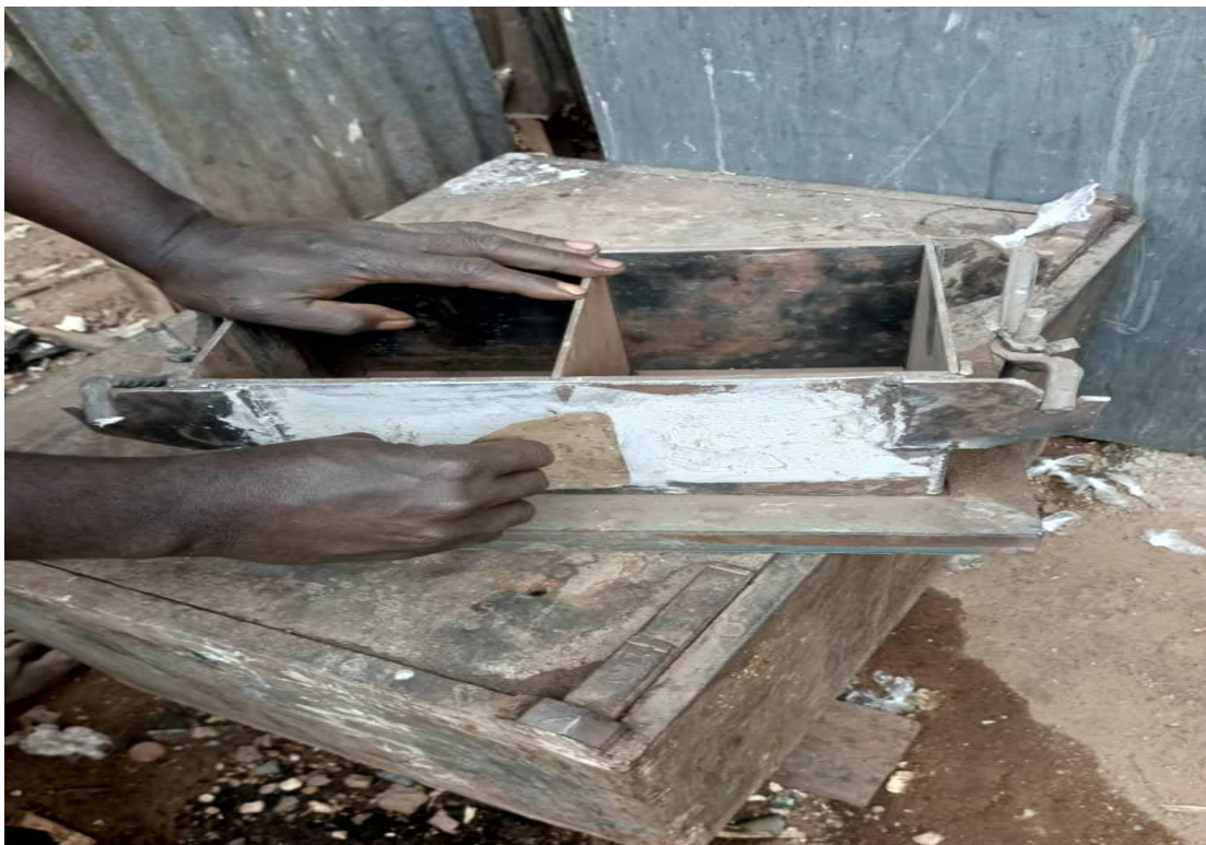
Plate 5: Body filling (puttying) after filing a dual cell metal concrete mold.
