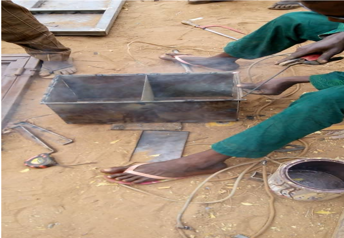
Plate 4: Connection of member Plates (Welding)
