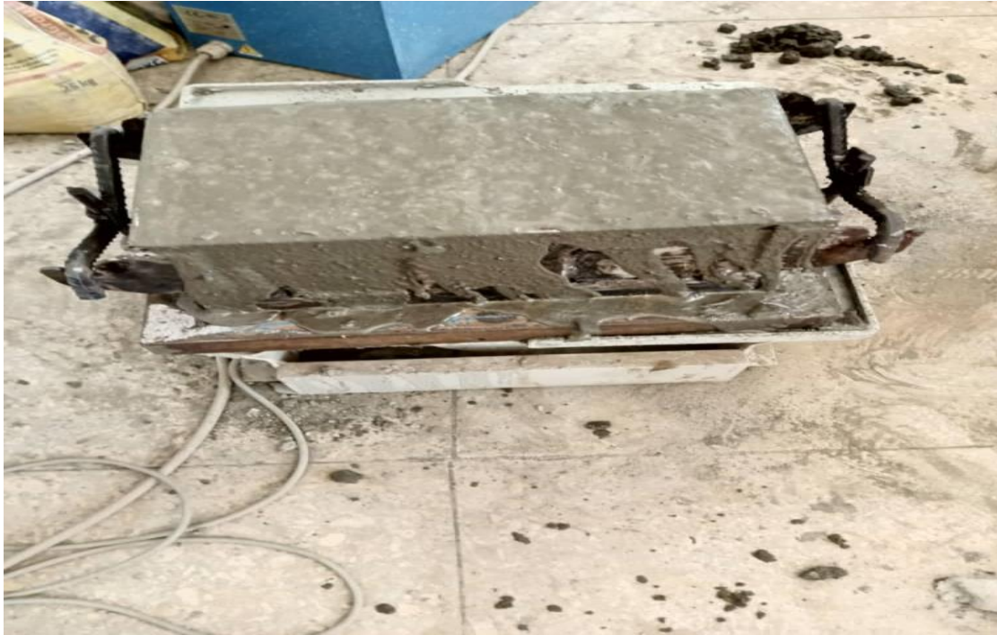
Plate 10: Compaction of concrete using a vibrator fitted with the fabricated mold to produce a cube.
