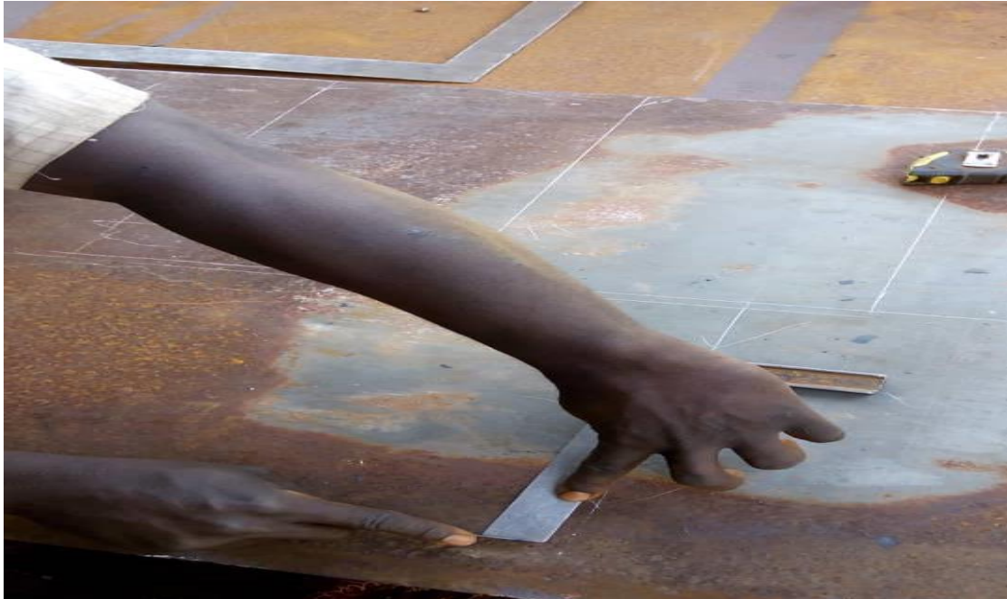
Plate 2: Marking out of members
