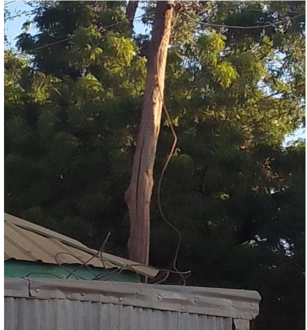
Figure 6. Service cable dropped on zinc
