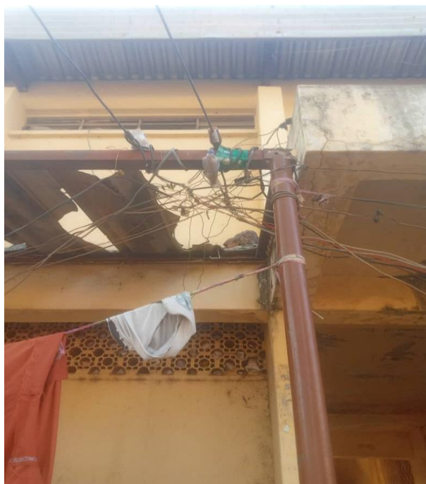
Figure 9. PVC Cables exposed to sun, rain and not exposed. Well arranged.
