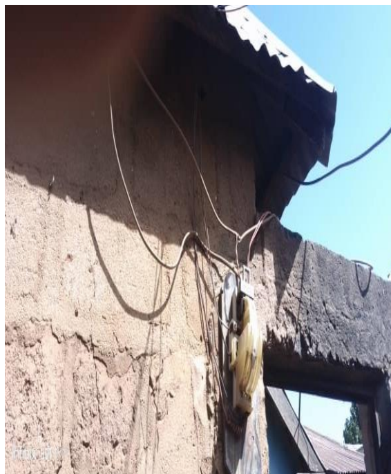
Figure 10. PVC Cables and control switch to sun and rain.
