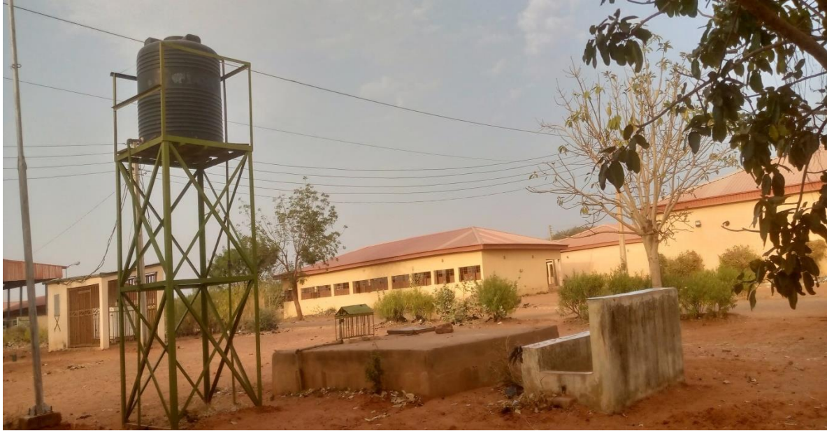
Plate 1: The Overhead Tank and the Reservoir that serve it Water
