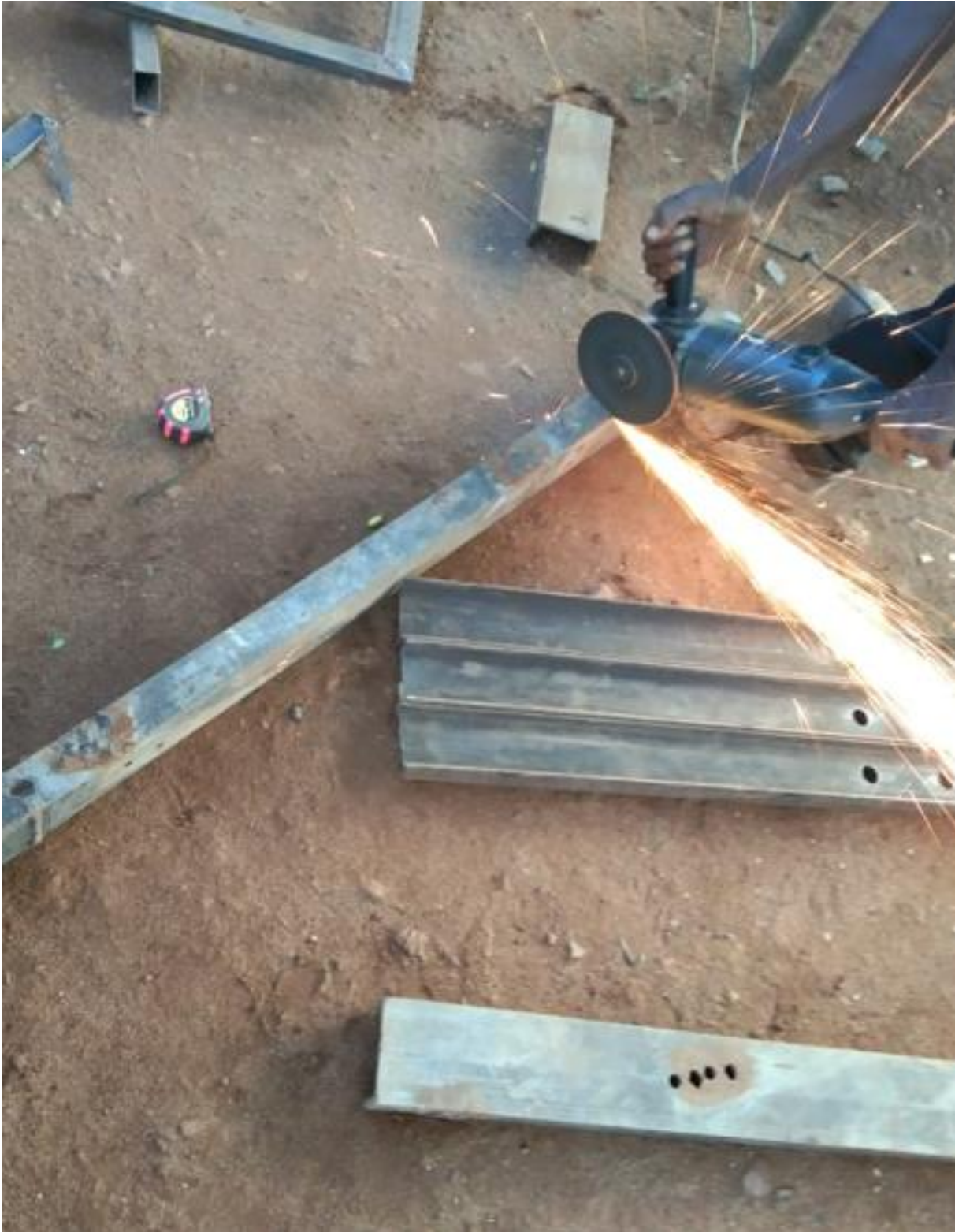
Slide 3: Fabrication of the main frame of the hydraulic press
