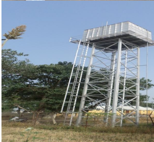
One of the Node and the overhead reservoir (Tank)
